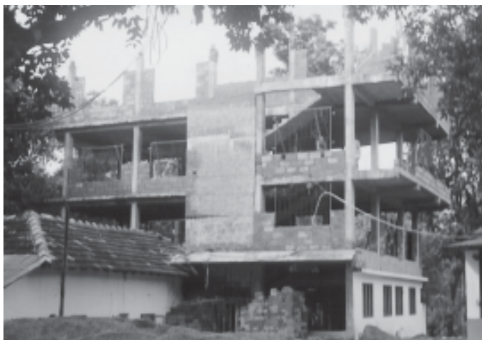
Photos: Above and upper left show the Phase One construction.
